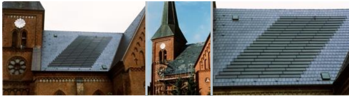
Church's roof covered with photovoltaic roof tiles, optimised array shape
