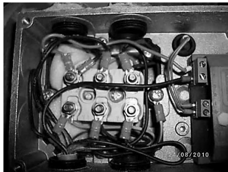
Three phase motor terminal plate
